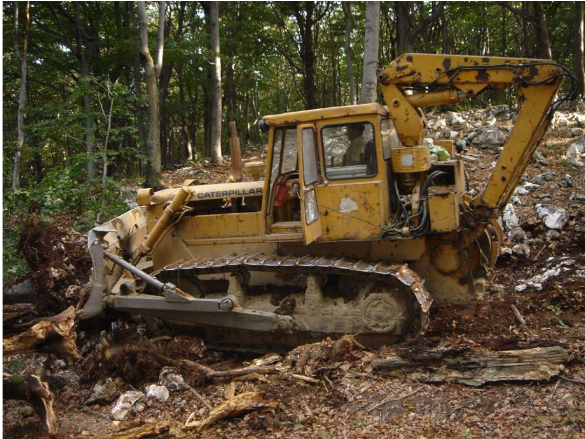
Figure 2. Caterpillar CAT D6 bulldozer, property of the "Grujić" company from Kučevo in action
