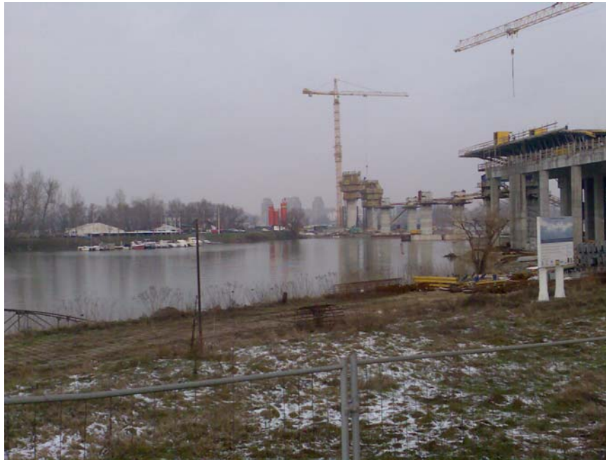
Figure 6. New Sava Bridge in construction (Photo R.Nevenic, 21. January 2010.)
