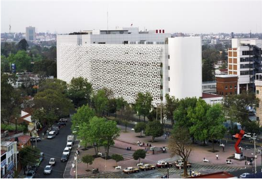
Figure 4. The façade of Manuel Gea González Hospital is said to negate the effects of up to 1,000 cars a day (image courtesy of Elegant Embellishments).
